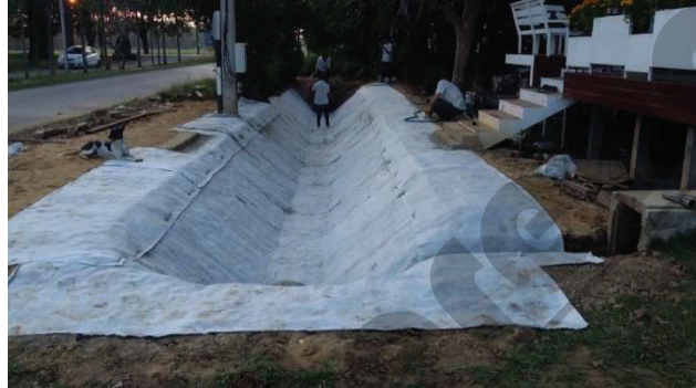
Figure 1 Farm ditch lining with concrete fabric
