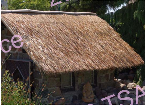
Figure 1. Vetiver roofing.
