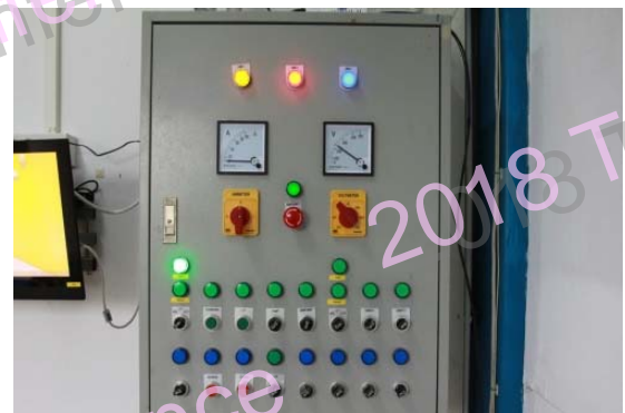
Figure 3 Controller board of TSBC Photo-Period House which design and built by Thailand Sugarcane breeding Center
