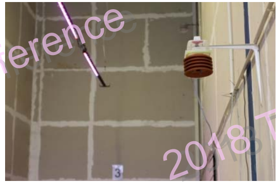
Figure 2 Electricity system for control day length, air condition system for temperature control and fogging system for humidity control in each compartments of TSBC PhotoPeriod House
