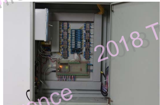
Figure 2 Electricity system for control day length, air condition system for temperature control and fogging system for humidity control in each compartments of TSBC PhotoPeriod House
