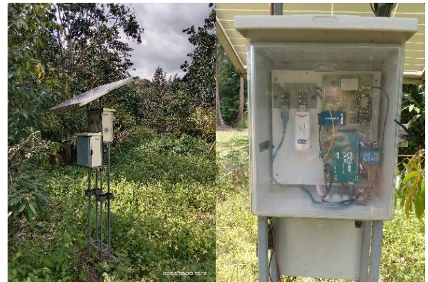
Figure 4 Equipment for recording environmental data in Thai cardamom plot.
