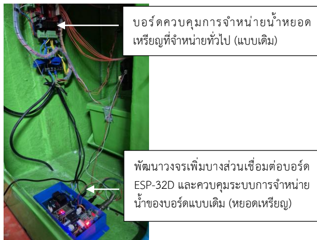
Figure 3 The ESP-32D board interfaces with the original board to control the water vending machine system.
