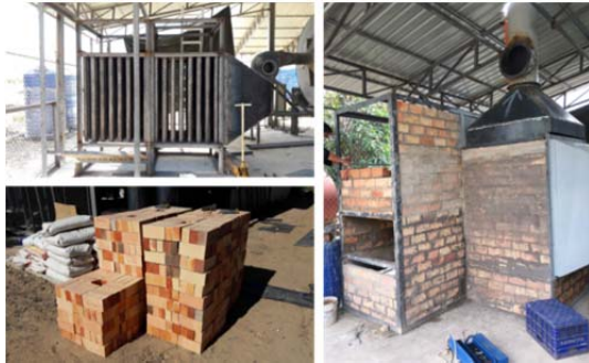
Figure 5 Fabrication of biomass furnace with heat exchanger.
