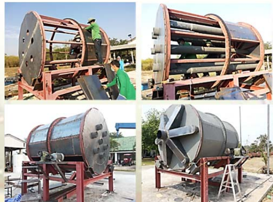
Figure 4 Fabrication of hot air duct of rotary dryer.
